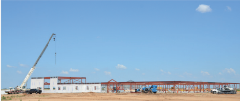
NEW FACILITY CONSTRUCTION SITE ON AUGUST 12
